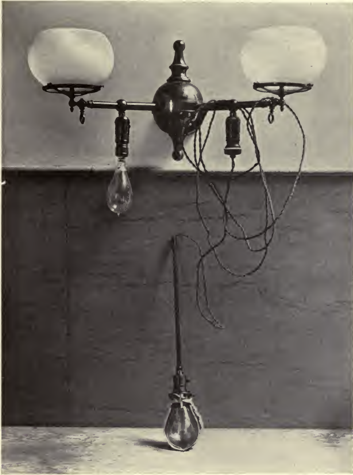
FIG. 19.—ELECTRIC DROP-LIGHT FOR USE IN ABDOMINAL OPERATIONS, CONNECTED WITH HOUSE CIRCUIT.
